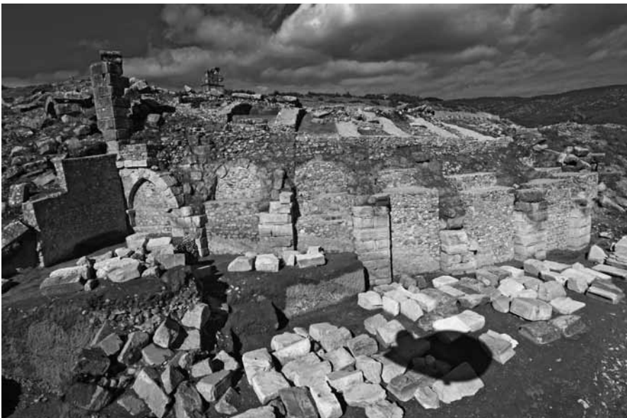
Fig. 9 Sphendone vaulted arch support for south-eastern two-storey retaining wall.
