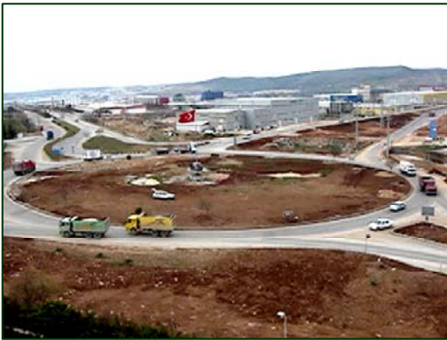
(Current view of Başbıran intersection) [d]
