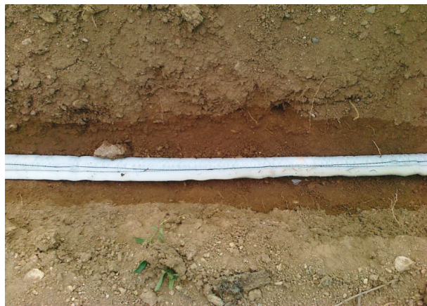
Figure 2. Uniform water transfer in the subsoil capillary irrigation method.
